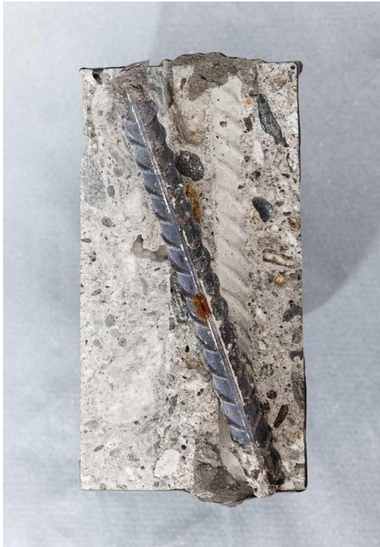
The combination of concrete and steel is hard to beat: even large reinforced concrete structures like bridges and tunnels are stable and durable.
